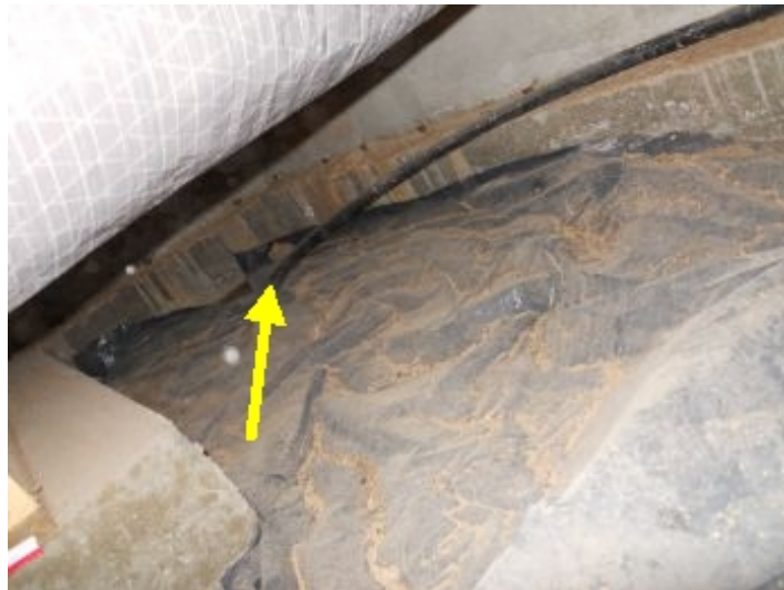
Main water line coming under foundation at NW corner
